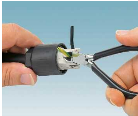
2. Cut the ends of the litz wires flush
